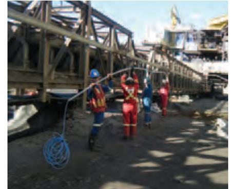
**Laying out the Shape Accel Arrays prior to installation in the MSE wall**
